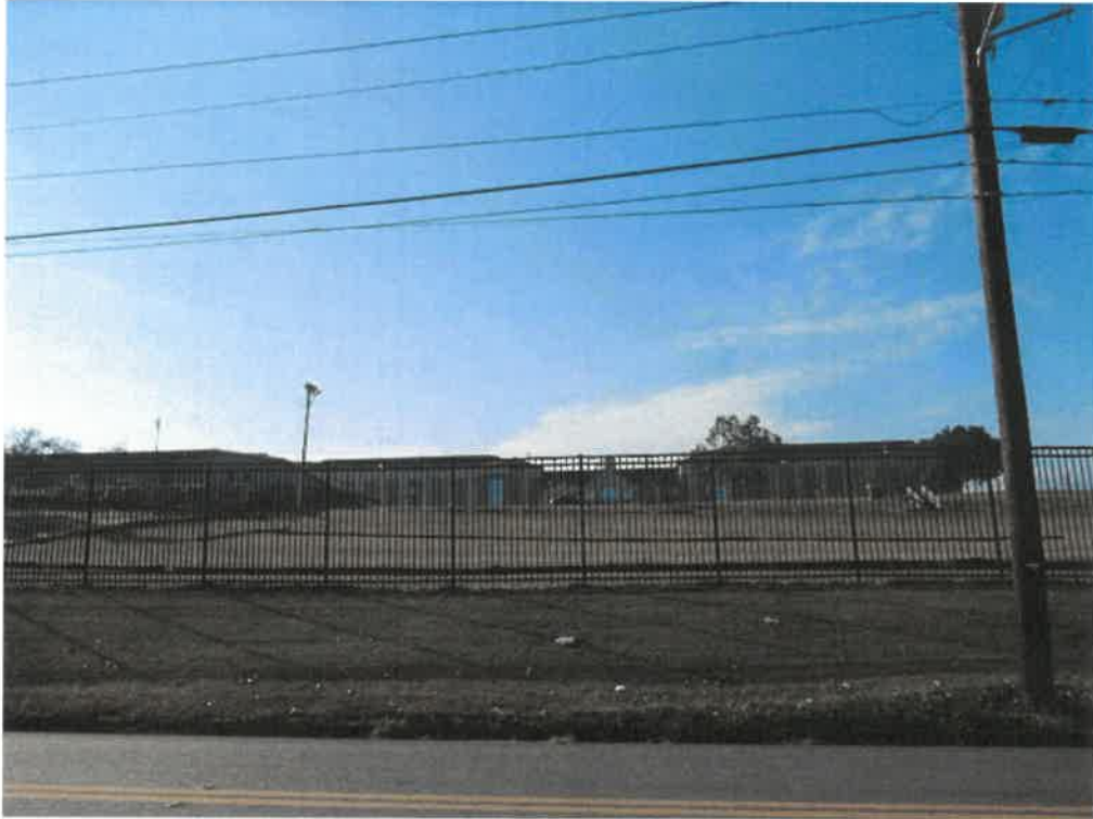
REAR VIEW OF FAMU ACROSS THE STREET
